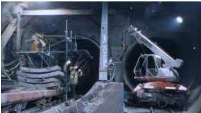
CX-8T – Underground on the Heathrow Express project lifting 1 Tonne tunnel segments into position at a radius of 6.5m with boom at 10m, from adjacent rail position. ▲
