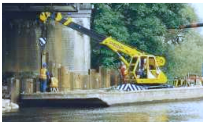
▲ Afloat on the River Avon, a CX-8T works installing Interlocking sheet piling under the low headroom of a mainline London/East Coast railway bridge.
