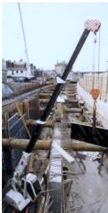
CX-3T ▲ Air-lifted onto sluice gate headings for Shuttering & Formwork duties at Cardiff Barrage
