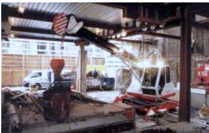
CX-8T – Working under low headroom in Savile Row, London ▲
