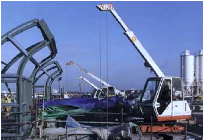
CX-3T ▲ Air-lifted onto sluice gate headings for Shuttering & Formwork duties at Cardiff Barrage
